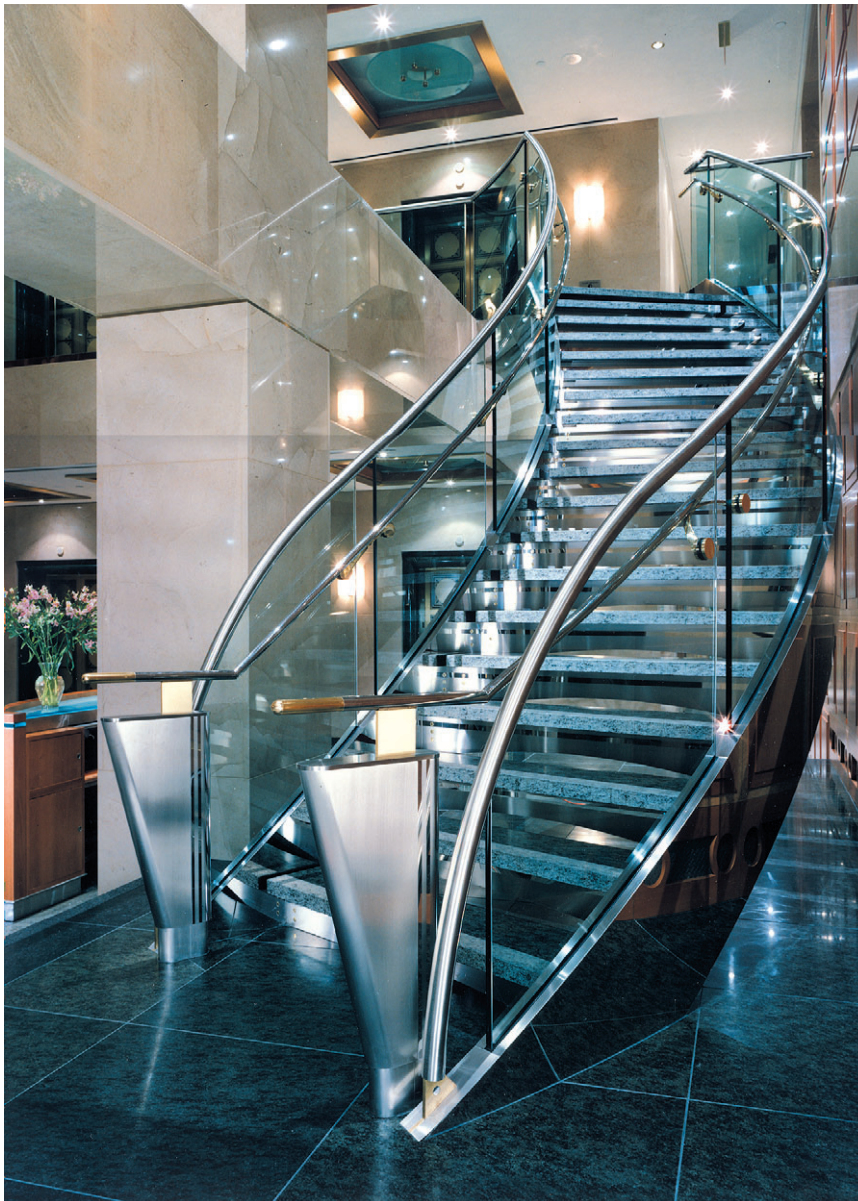
Monumental st. stl. staircase with mirror polished st. stl. stringers and guardrails and curved tempered glass
