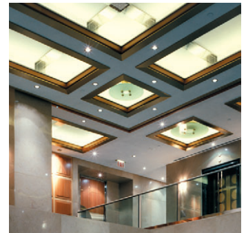
Brass framed ceiling with frosted circular glass light fixtures
