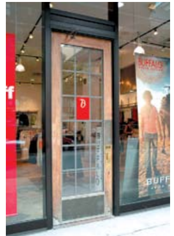
White oak side door and curtainwall
