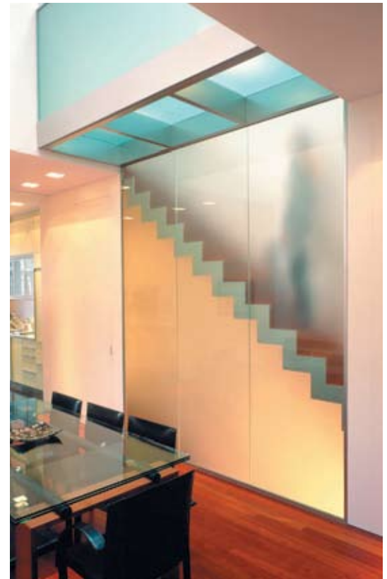
Stainless steel and glass bridge and staircase with fiber optic accent lighting
