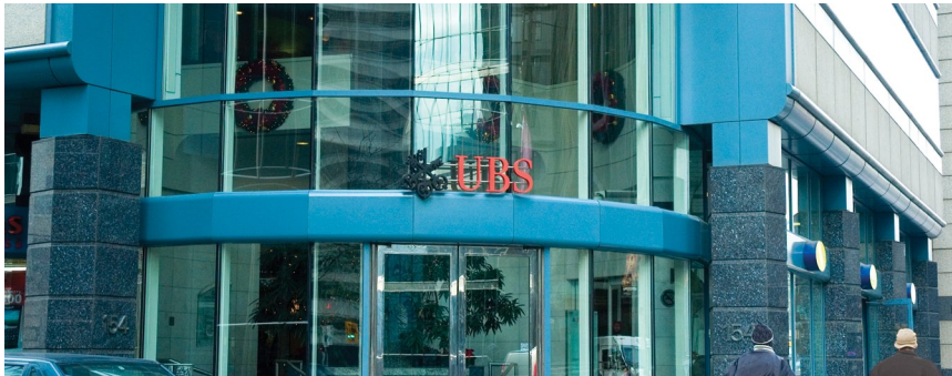
Prominent business identification sign mounted to building's structural steel
