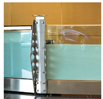
Modern fasteners and framing
