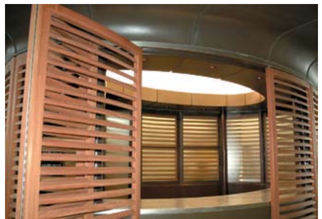
Front doors of kiosk, made of solid jatoba, revealing stainless steel counter
