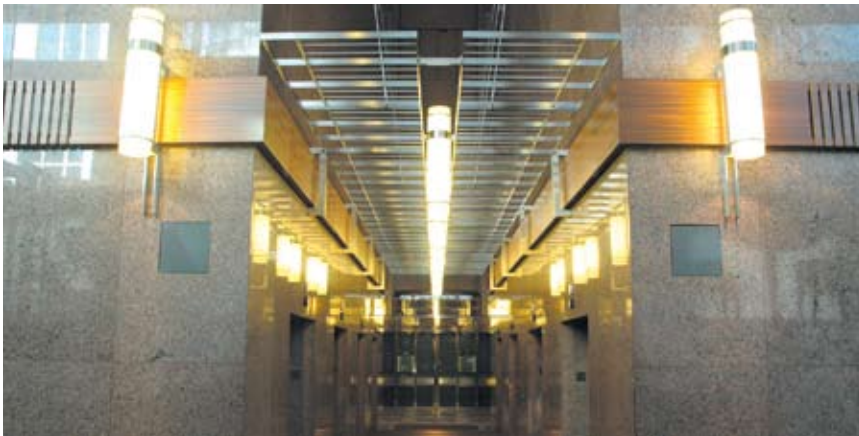
Overhead elevator lobby canopy with light fixtures
