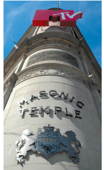
Letters and crest installed on curvature of building
