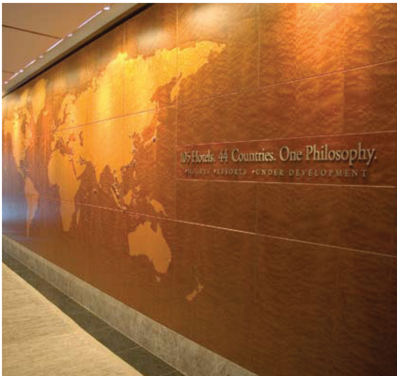
The History Corridor World Map Wall in Pomelle Makore Veneer with Maple Inlay and Stainless Steel Graphics
