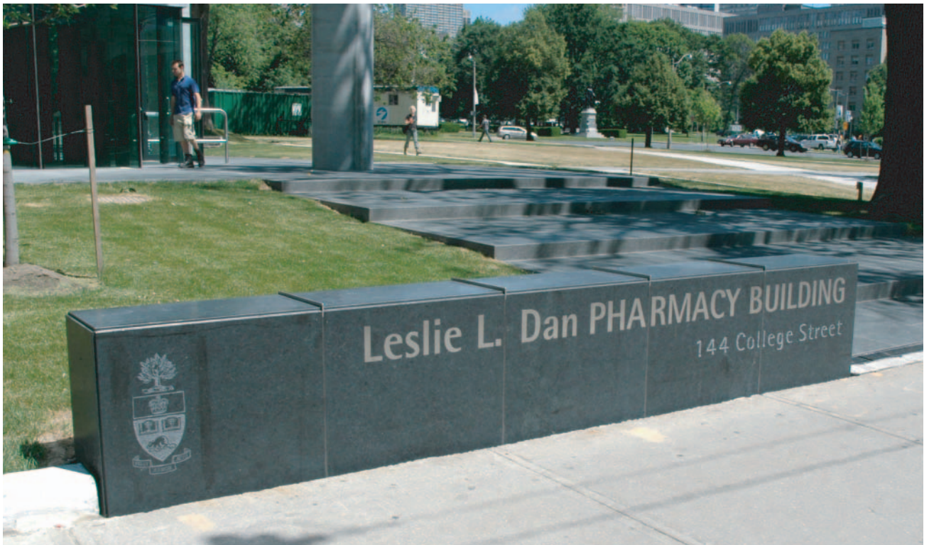
Precision carved granite and incised waterjet cut st. sl. lettering
