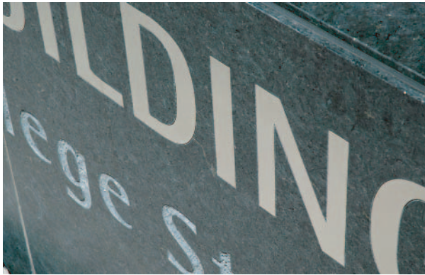
Waterjet cut, brushed st. sl. graphics incised into 1-1/4" thick granite
