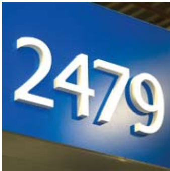
Precision cut graphics on aluminum cladding
