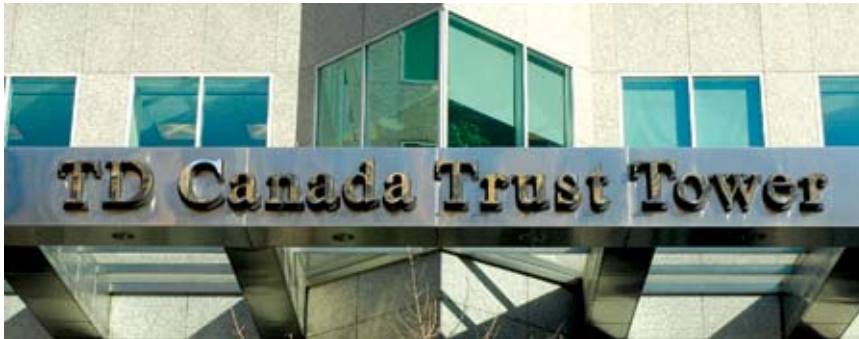
Dual layer, mirror polished stainless steel water-jet cut graphics on painted backing, mechanically mounted
