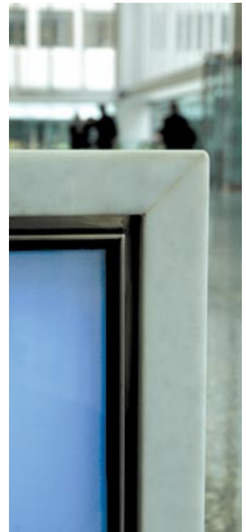
Detail of the marble finishing & joinery
