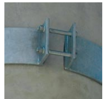
Solid, bolted lap joint connection
