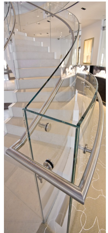
Detail of the custom handrail
