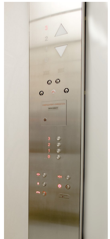
Stainless steel control operating panel (COP)
