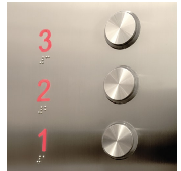
Detail of the COP with braille embossing
