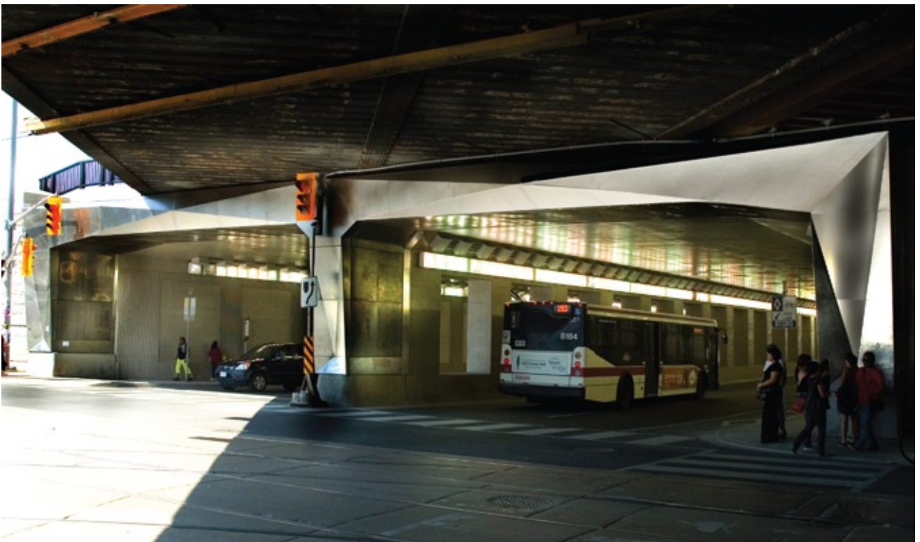
The Dufferin Street Jog portal with stainless steel portal cladding.
