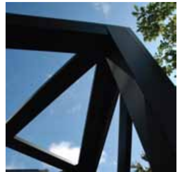
Detail of an upper corner connection
