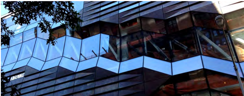
The patinated muntz paneling where it meets and joins with the glazing on the building envelope
