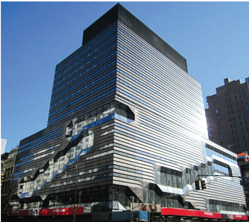
The New School at 65-5th Avenue with completed cladding of the building envelope
