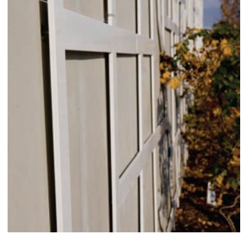
Mechanical fastening with 1/4" relief from wall
