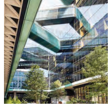
Detail of paneled bridges and trim
