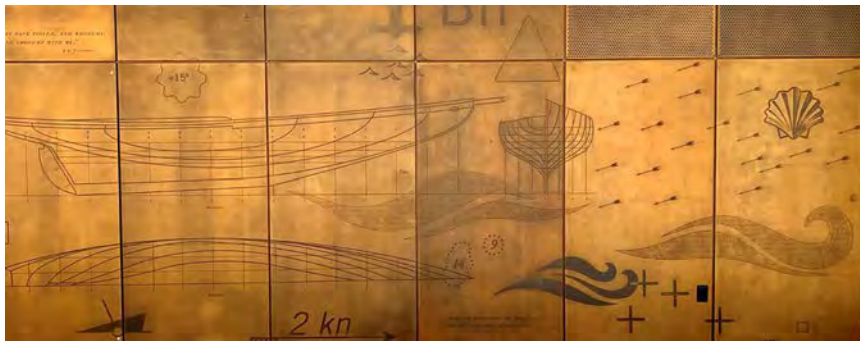
Patinated Muntz panels with etched artwork spanning across multiple panels
