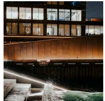
Curtain wall panels along the steps into the water
