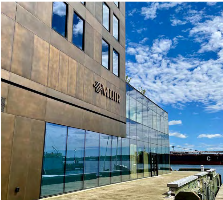
Patinated curtain wall panels at the entrance to the Muir Hotel at Queen's Marque
